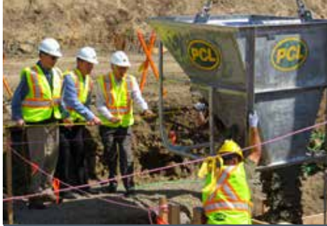
Left: Workers pour concrete at a new hospital and health centre in Burns Lake, B.C. Photo courtesy of B.C. Northern Health Authority.
