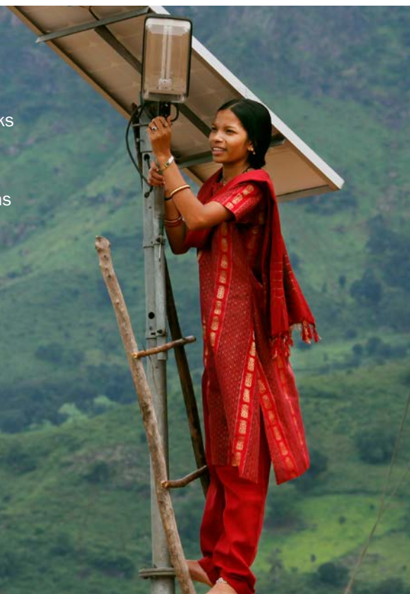
Photo: Meenakshi Dewan tends to maintenance work on the solar street lighting in her village of Tinginaput, India. Huge pylons run across these hills, supplying power to the big cities – but rural areas like this are not connected to the main grid.
