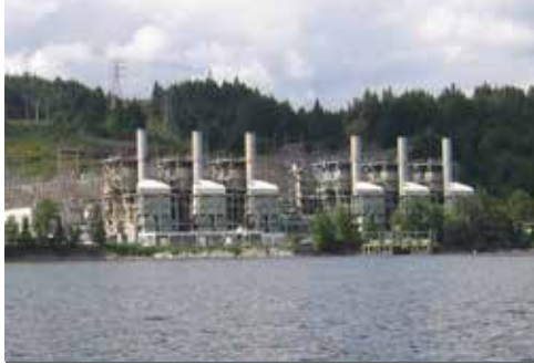
Left: The Burrard Generating Station is maintained by BC Hydro to generate electricity from natural gas. Photo: Niall Williams, Flickr.
