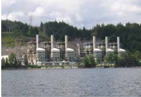
Left: The Burrard Generating Station is maintained by BC Hydro to generate electricity from natural gas. Photo: Niall Williams, Flickr.
