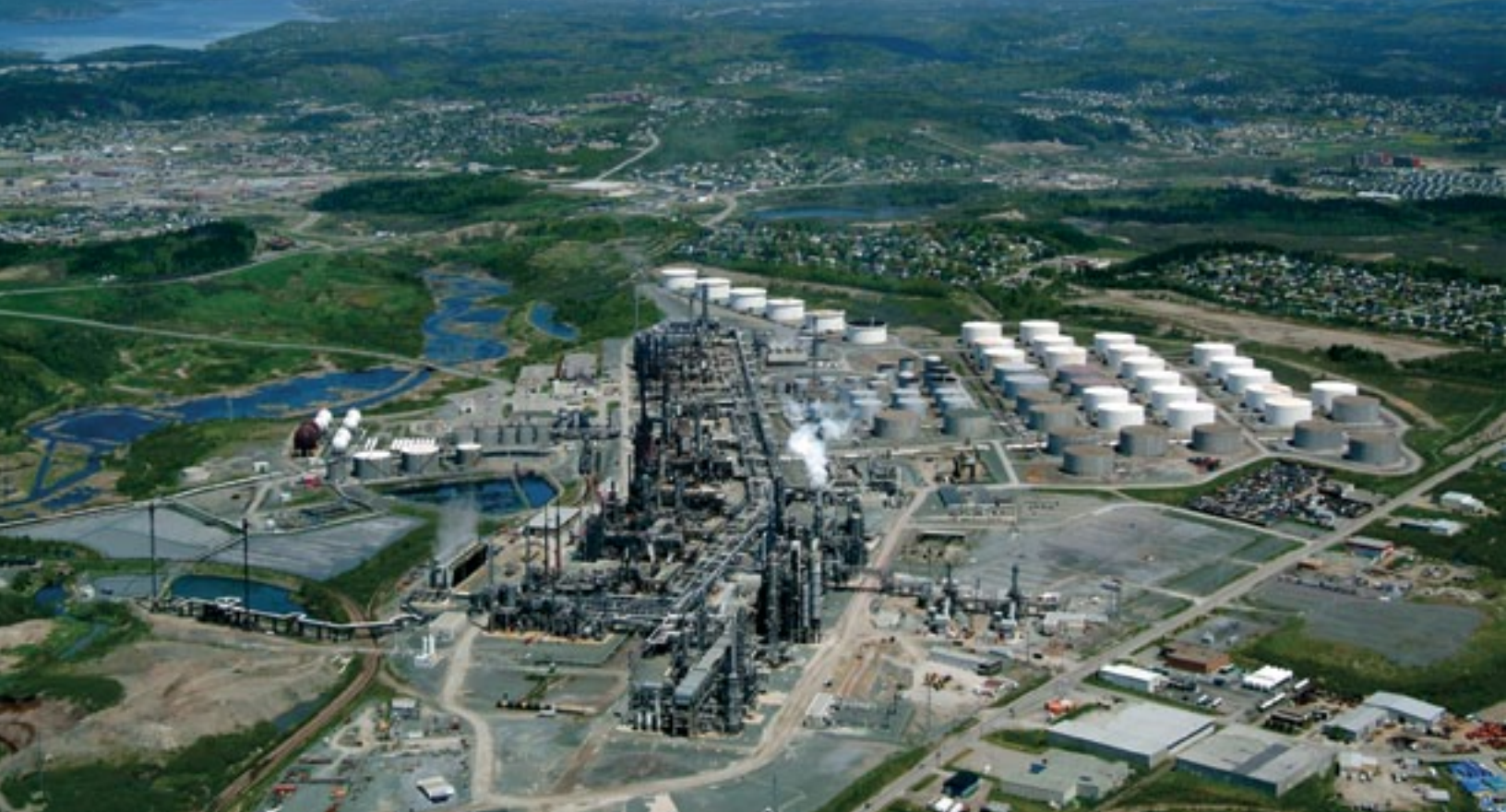
The Irving refinery in Saint John is the largest in Canada, with a capacity of 300,000 barrels of oil per day. Nearby Saint John Harbour is the deepest on the east coast of North America. Irving Oil photo
