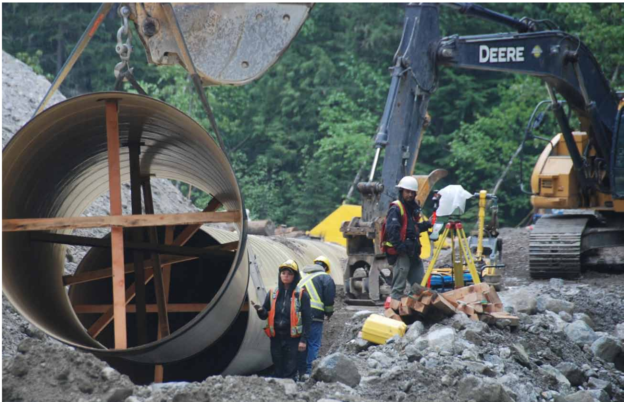
First Nations workers assemble a section of penstock for the Kwoiek Creek run-of-river hydroelectric project. Photo: Innergex Renewable Energy.
