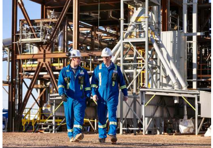
Enerkem's waste-to-fuel facility in Edmonton
